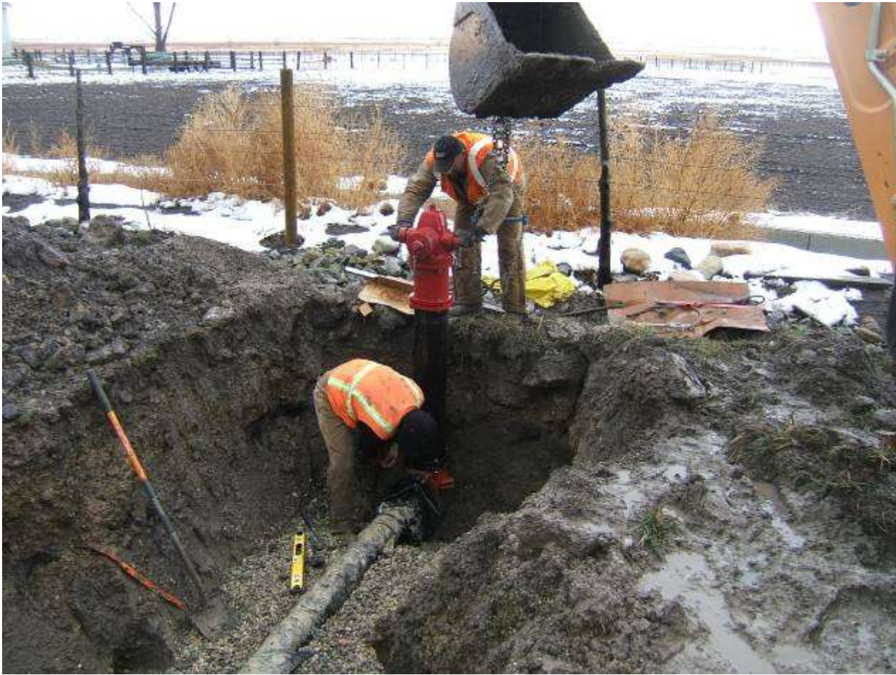
Installation of hydrants along Highway 38 in Harper Ward – November and December 2010
