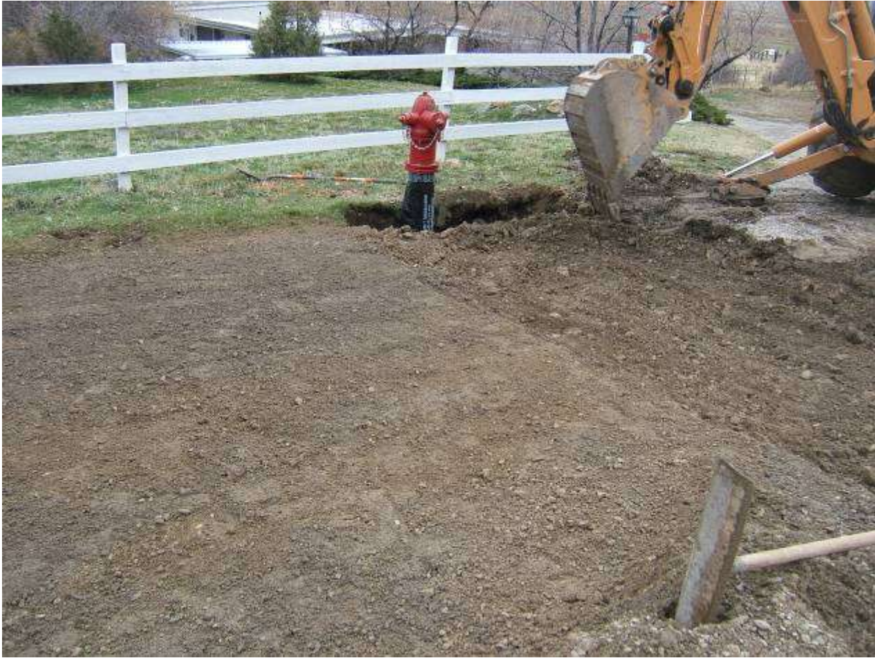
Backfill and grading around newly installed hydrant – December 2010
