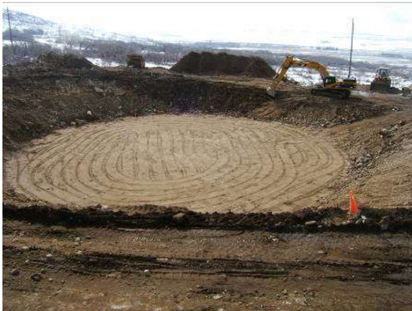
Completed grading & compaction for Reservoir 2009
