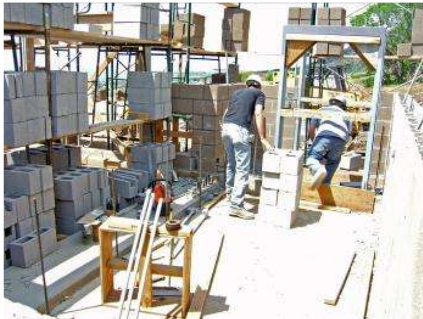
Masonry construction beginning on the pump station
