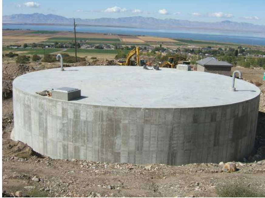
1 M Gallon Reservoir - October 2009
